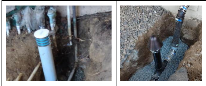
Above are two the two kinds of backflow prevention devices. If your sewer isn't equipped with one of them, you are at risk for having sewage flow into your house in the event of a sewer backup.
