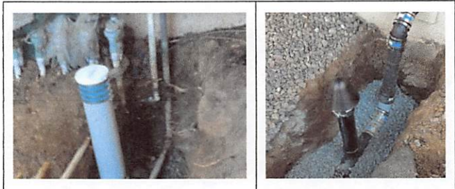
Above are two the two kinds of backflow prevention devices. If your sewer isn't equipped with one of them, you are at risk for having sewage flow into your house in the event of a sewer backup.
